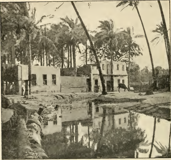
FIG. 7.—The canal forming a shallow pool in the village square.
